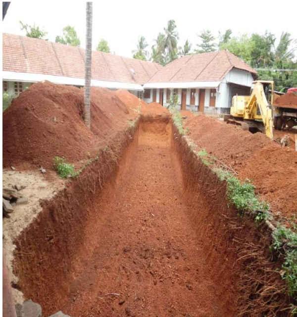
2. JCB digging up soil for foundation
